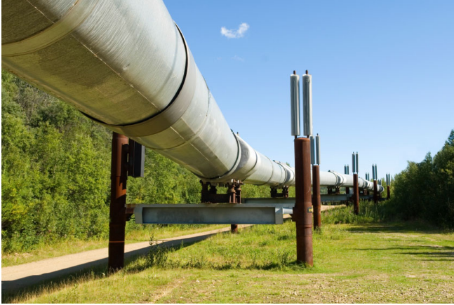
Figure 7: The Pipeline Insulation model in the application library simulates the effect of viscous heating on the cooling and transport properties of oil in a pipeline.
