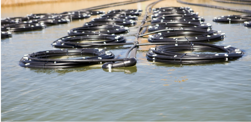
Figure 1: A sled carrying pipe coils shown before the system is submerged.
