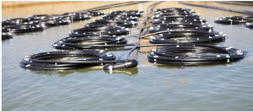
Figure 9: A sled carrying pipe coils shown before the system is submerged.
